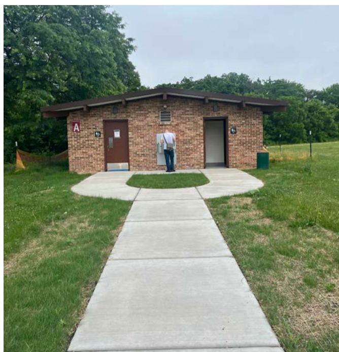
New Accessible Restroom Path at Busse Woods
