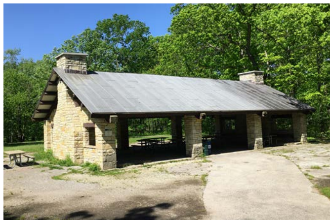
Shelter Repair at Harms Woods
