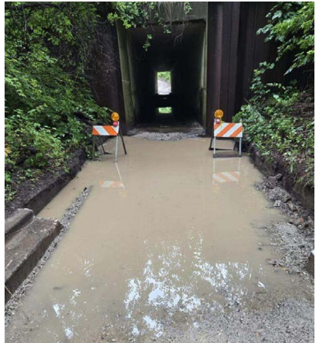
Thorn Creek Trail Repair
